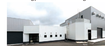
Material MBR Building / Data-Driven Technology Research Building
